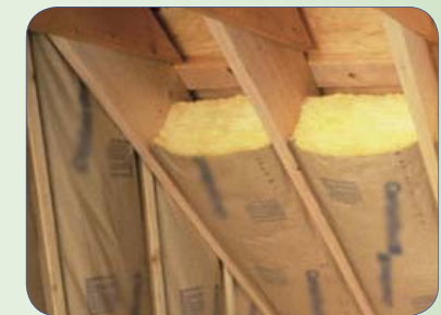
High levels of insulation in walls and roof. Keeps warm in winter, cooler in summer, reducing reliance on finite energy resources.
