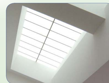
High level of natural light. Reduces reliance on electric lighting.
