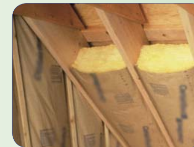
High levels of insulation in walls and roof. Keeps warm in winter, cooler in summer, reducing reliance on finite energy resources.
