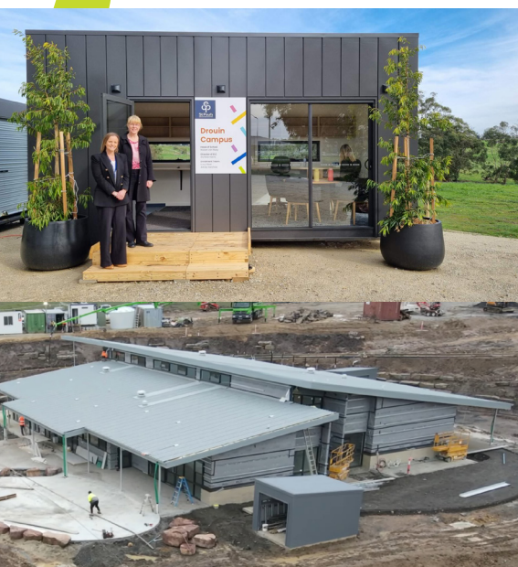
Drouin site office and ELC in progress.
